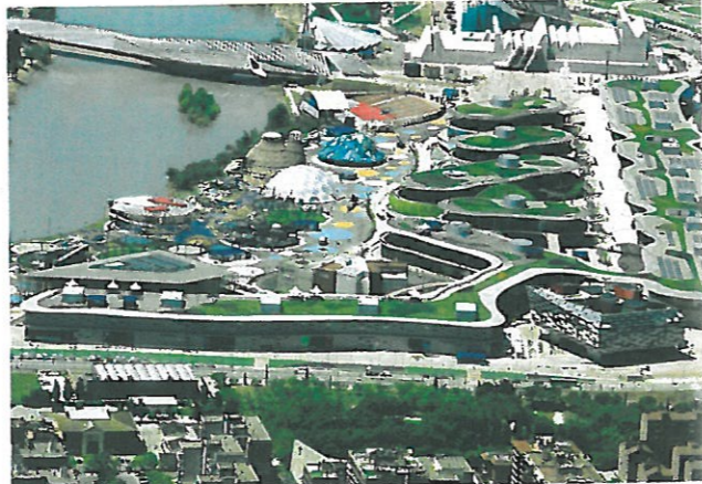
Fig 3. Aerial view of the whole green roof.
